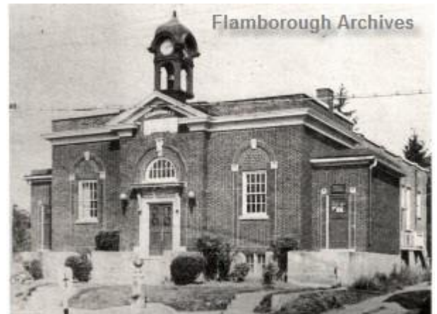
The Waterdown Memorial Hall after completion in 1922
